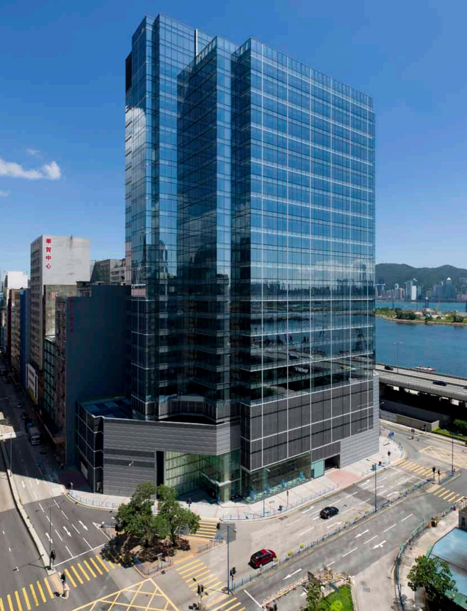
**These pages** The many mullions, transoms and spandrels that make up the facade of One Harbour East have been arranged in a tartan-like pattern inspired by the famed Burberry print. The staggered facade responds to site geometry, as well as providing increased corner office space.
